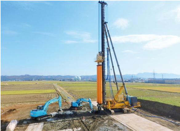
Ground improvement project for road construction (Onoda Chemico Co., Ltd.)
