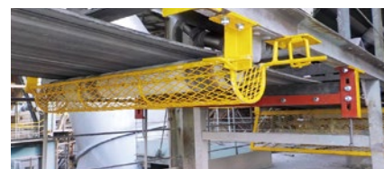
Safety cover for self-aligning return roller Registration No.: 03235767 (February 3, 2022)
