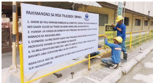
Posting of warning to drivers (Taiheyo Cement Philippines, Inc.)
