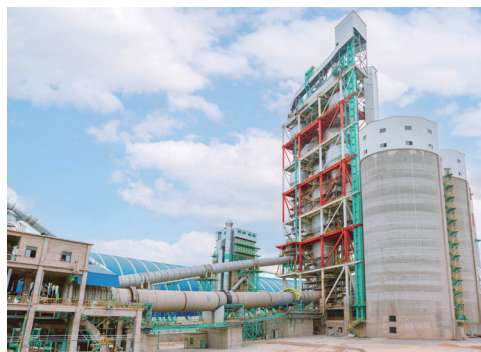
Taiheiyo Cement Philippines, Inc. Cebu Plant (Philippines)
