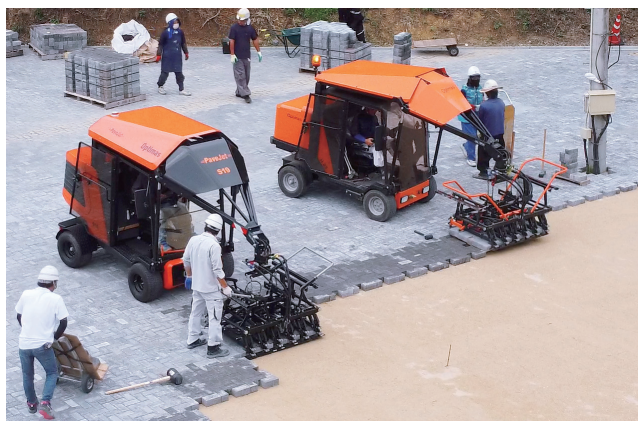
German-made IL block dedicated laying machine
