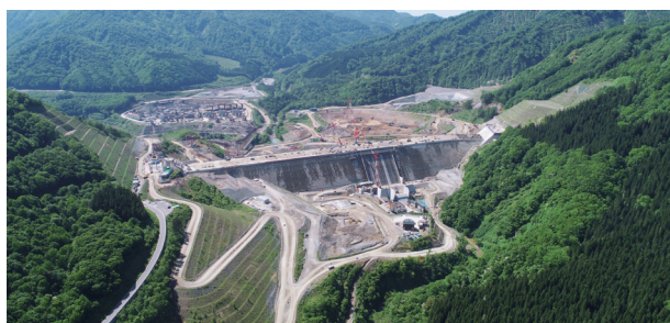
Naruse Dam construction site (photographed in May 2024)
