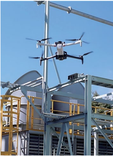
Equipment inspection using drones
