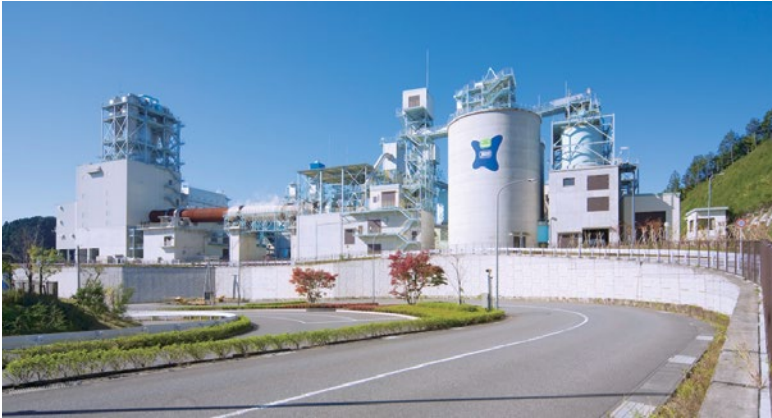
Tokyo Tama Ecocement Facility (Overall View)
