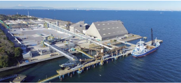
Minamisode Aggregate Yard
