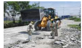
Employees repairing a road
