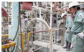
Providing safety guidance at a ready-mixed concrete plant
