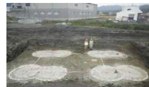
Extent of ground improvement
