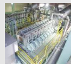
Gas engine at the Kumagaya plant
