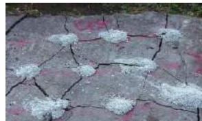
Cracks generated after BRISTAR has been activated
