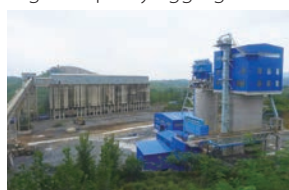
Reconstructed aggregate plant for reducing environmental impact
