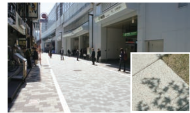
Using "Ocean Eco Cool" in road construction work near Kanda Station
