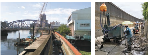
Using NJP-2way in seismic retrofitting for the flood barrier of the Sumida River
