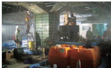
Seismic retrofitting work
