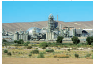
CalPortland Company, Oro Grande Cement Plant (U.S.A. Oro Grande)
