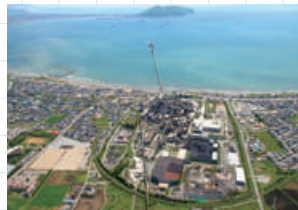
Taiheiyō Cement Corporation Kamiiso Plant
