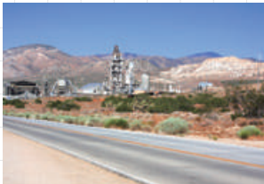
CalPortland Company, Mojave Cement Plant (U.S.A. Mojave)
