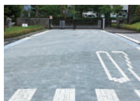
Paving blocks constructed for evaluation
