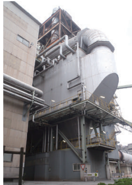
WHR power generation system (waste heat boiler on the kiln preheater system at the Kamiiso plant H-8)
