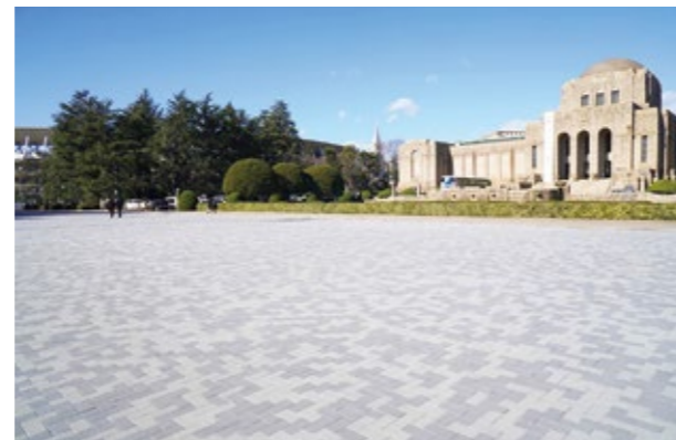
Thermalbarrier ILB laid in the plaza in front of the Meiji Memorial Picture Gallery in Jingu Gaien
