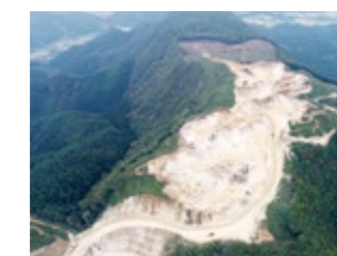
Horoshi area of the Ofunato Quarry
