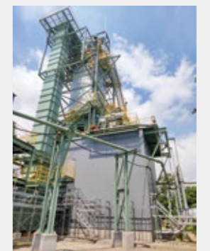
Kamiiso Plant Waste Plastic Receiving and Processing Facility
