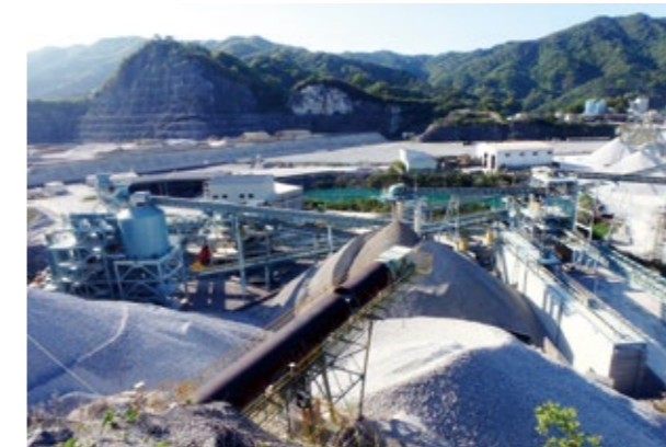
Aggregate classification plant (Shin-Tsukumi Quarry)
