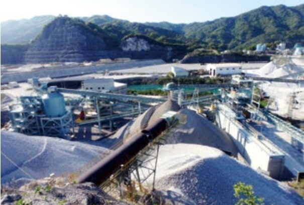
Aggregate classification plant (Shin-Tsukumi Quarry)
