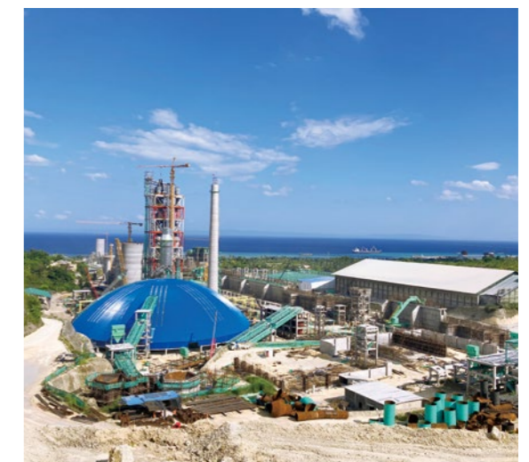
The renovation of the production line (Taiheiyo Cement Philippines, Inc.)
