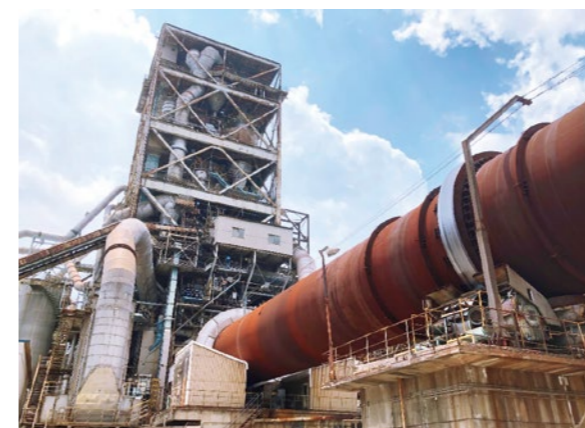
Fujiwara Plant No. 5 Kiln (installation of high-efficiency clinker coolers)
