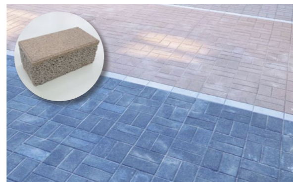
Trial laying of interlocking blocks manufactured with CARBOFIX cement Interlocking blocks manufactured with CARBOFIX cement were laid in a parking lot to confirm their applicability as paving blocks. Technology development is in progress to further expand their CO 2 reduction effect.
