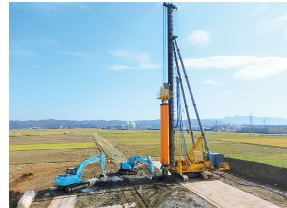
Ground improvement project for road construction (Onoda Chemo Co., Ltd.)
