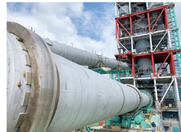
Renovation of production line (Taiheiyo Cement Philippines, Inc.)
