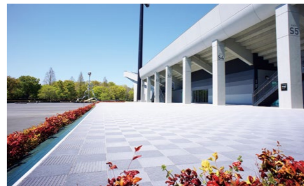
Construction example: Thermalbarrier ILB laid around the rugby field at Kumagaya Sports Culture Park, Saitama Prefecture
