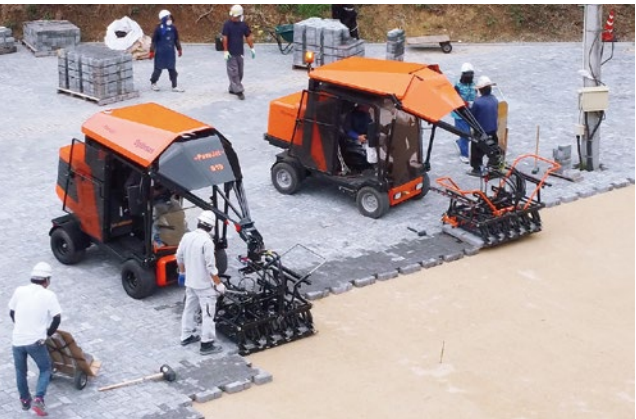
German-made IL block dedicated laying machine
