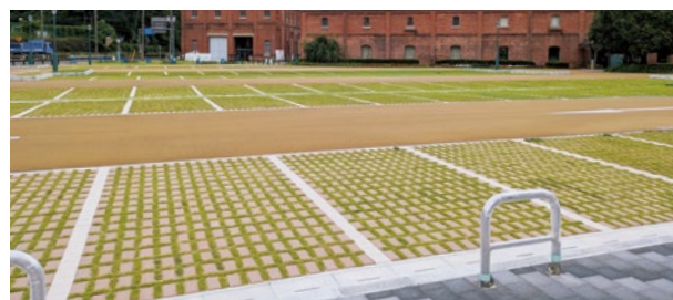
Planting grass between blocks mitigates the effect of the heat island phenomenon
