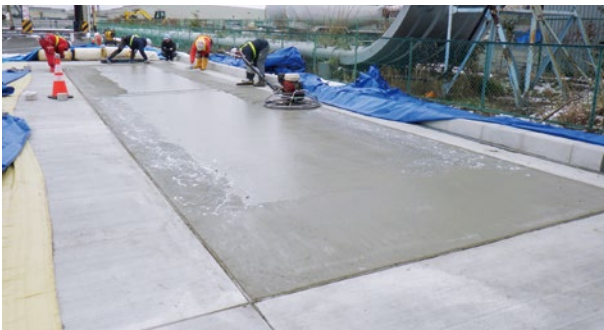
Test construction of a concrete pavement using CarboCatch slurry
