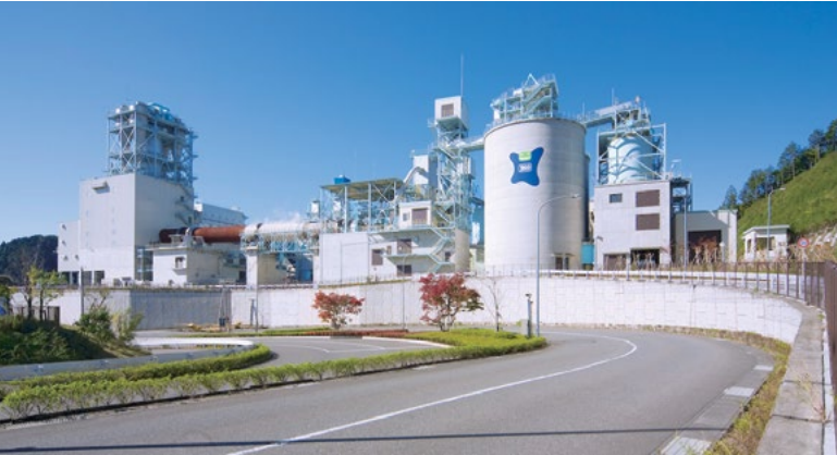
Tokyo Tama Ecocement Facility (Overall View)
