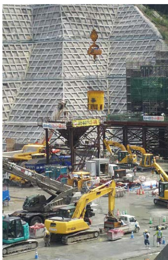
Yamba Dam Concrete Placing
