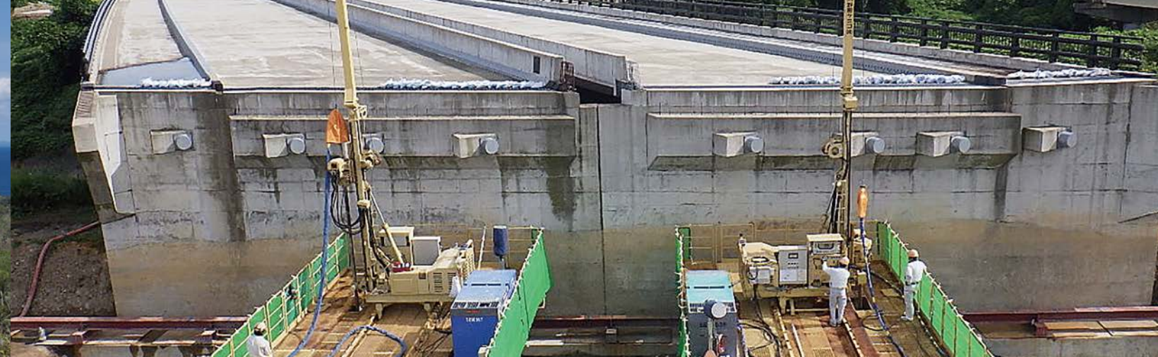
Ground improvement works (LDis-Dy Method) (Onoda Chemico)
