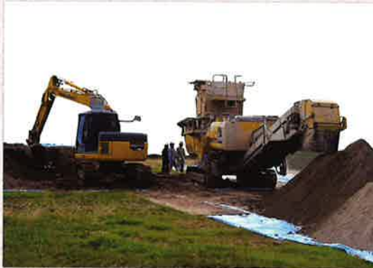
▲ Application using a self-propelled soil improvement machine (powder addition)
