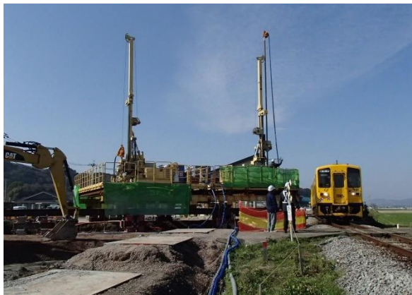
Soil stabilization project near a railway line using the LDis method
