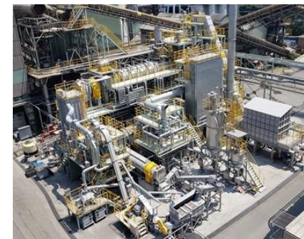
Facility using low-temperature embrittlement to recycle waste plastic that is difficult to process (Kawasaki Plant of DC CO., Ltd.)
