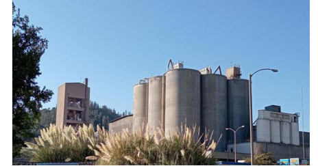
CalPortland Redding Plant (California, US)
