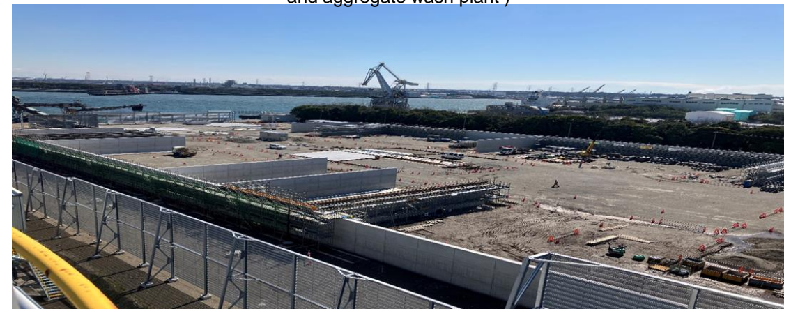
New Minamisode aggregate yard under construction (Sodegaura City)
