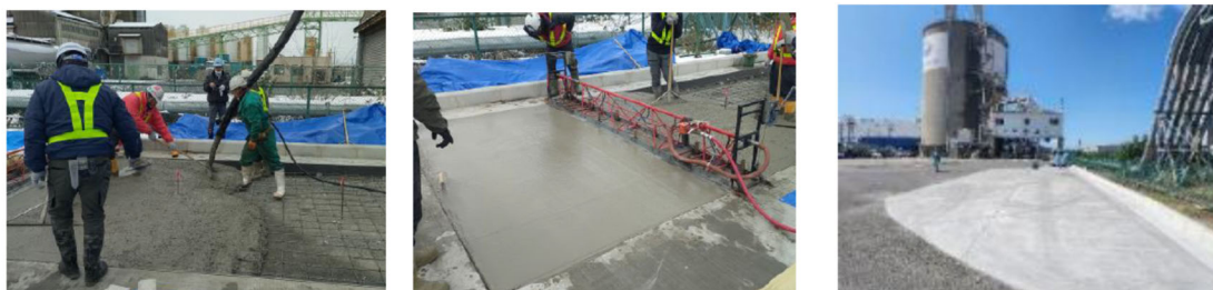
Figure 3. Situations of construction and service of pavement concrete using CARBOCATCH™ slurry.
