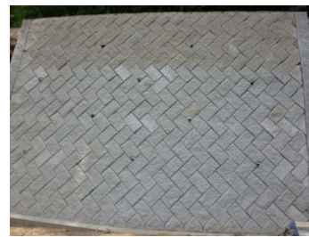
Photo 2: A slope restored with the low-carbon blocks
