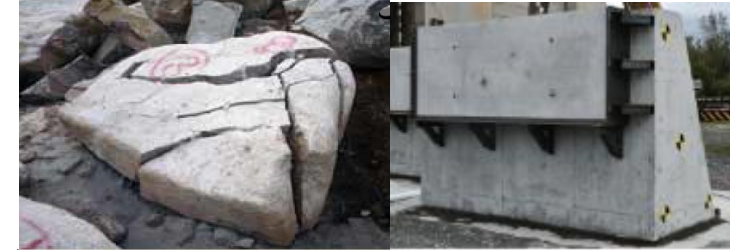
BRISTAR for crushing fallen rocks (non-explosive demolition agent)
