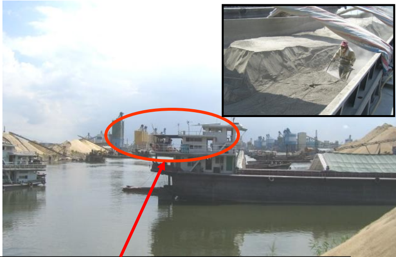
PFA Cement Fuyong/Silo Complex
