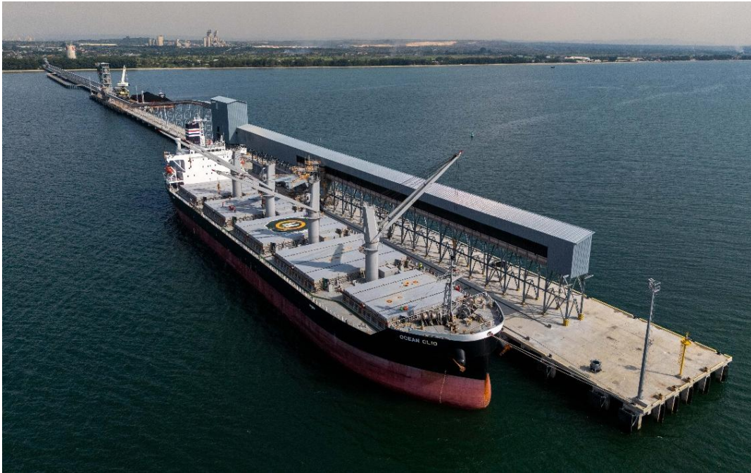
SBI's Tuban Plant: Export Jetty and Cement Carrier
