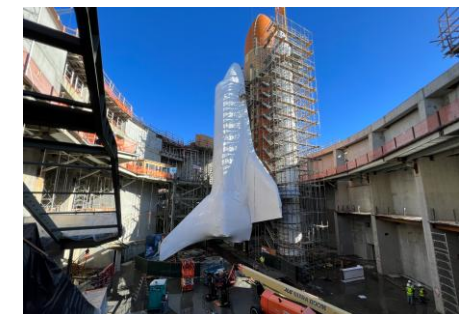
Delivery case of Type IL (Blended Cement) Used for a 17,000 cy concrete structure Inside The California Science Center (Los Angeles)
