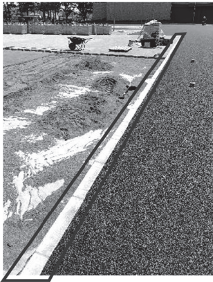
Fig.17 After construction (施工後の様子)
