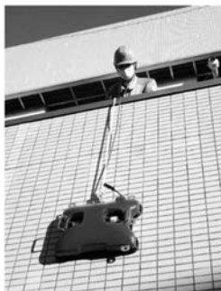
Wall Survey Robot
